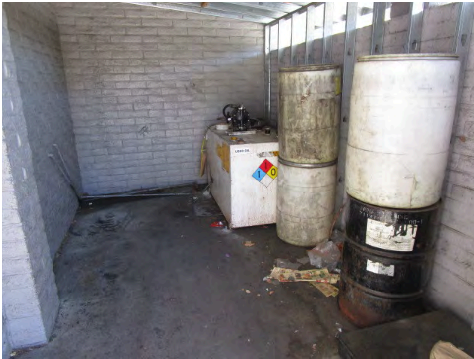
12. Enclosure at the southern end of the building
