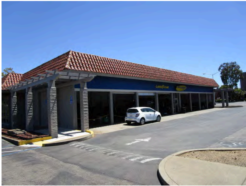
1. Western side of the subject property building
