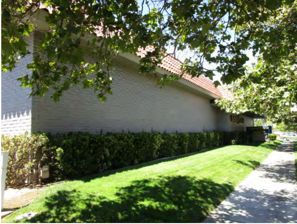
5. Eastern side of the subject property building
