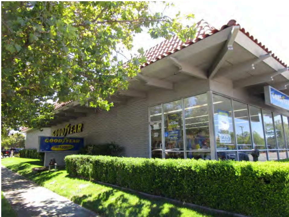
4. Eastern side of the subject property building
