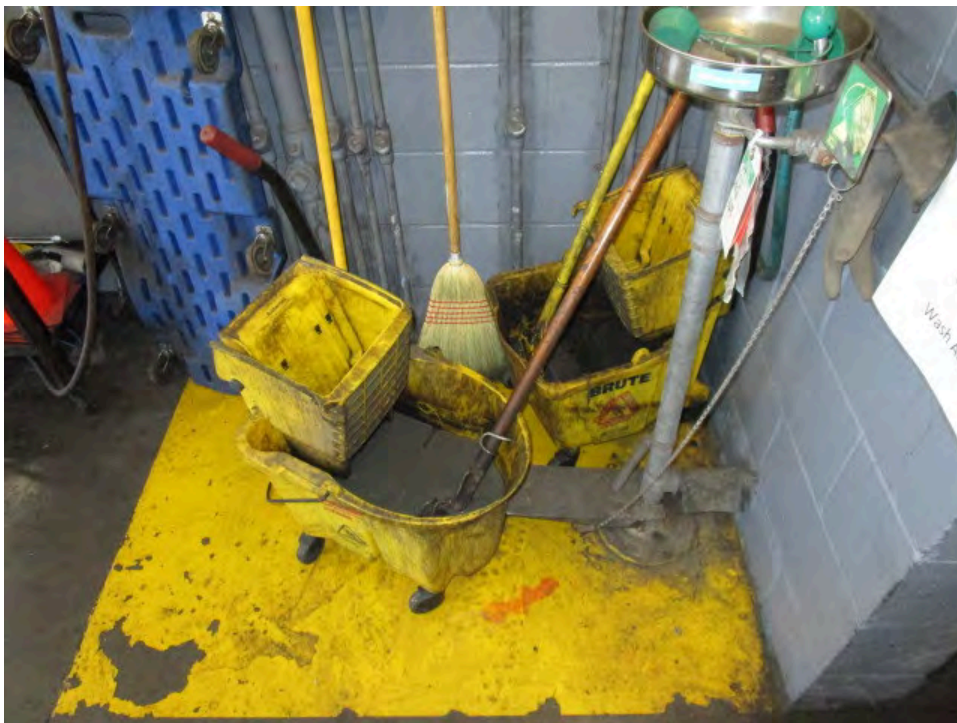
36. Mop buckets in the automotive service area
