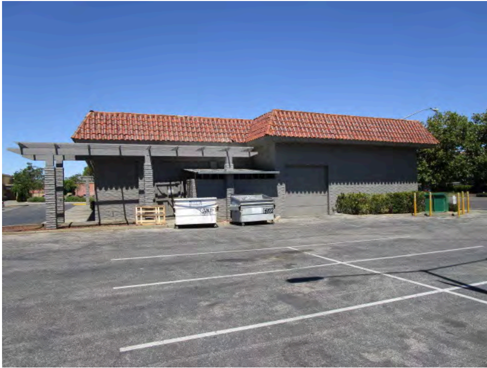
3. Southern side of the subject property building
