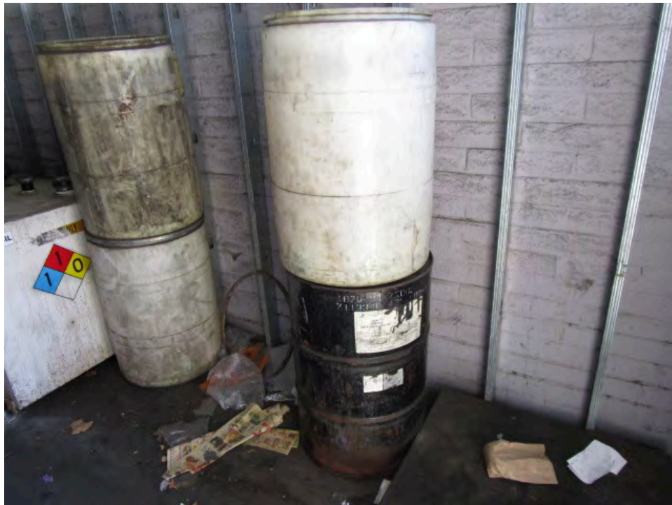
14. Empty drums and an anti-freeze drum in the enclosure on the southern side of the building
