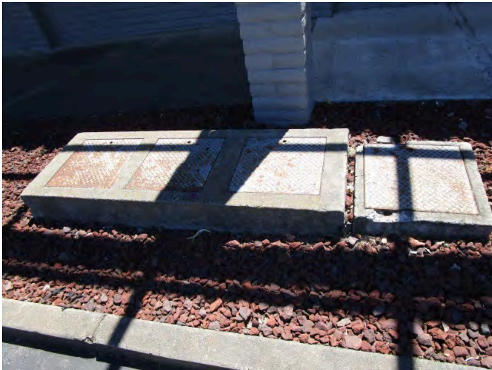
6. Clarifier adjacent to the northern side of the subject property building
