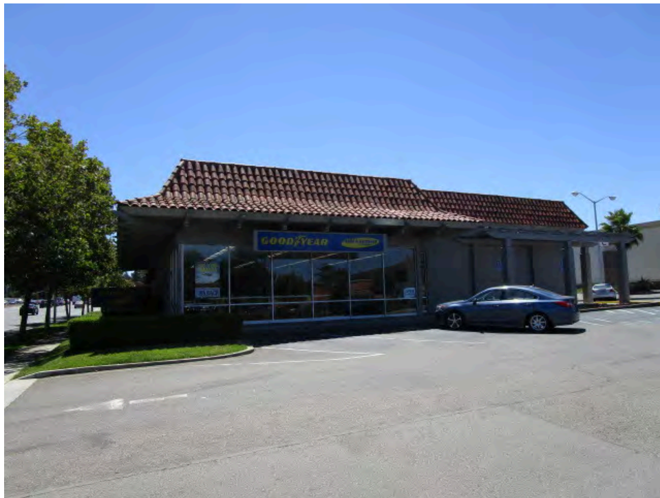
2. Northern side of the subject property building
