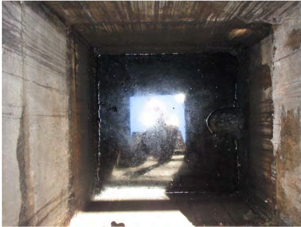
7. Interior of the clarifier
