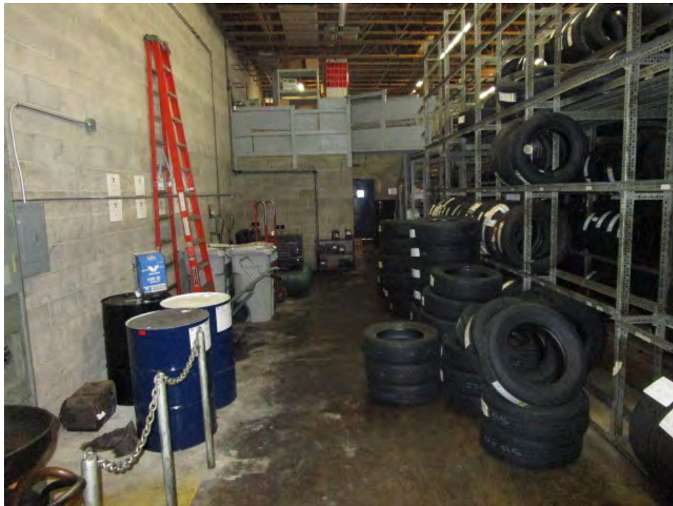
28. Overview of the store room
