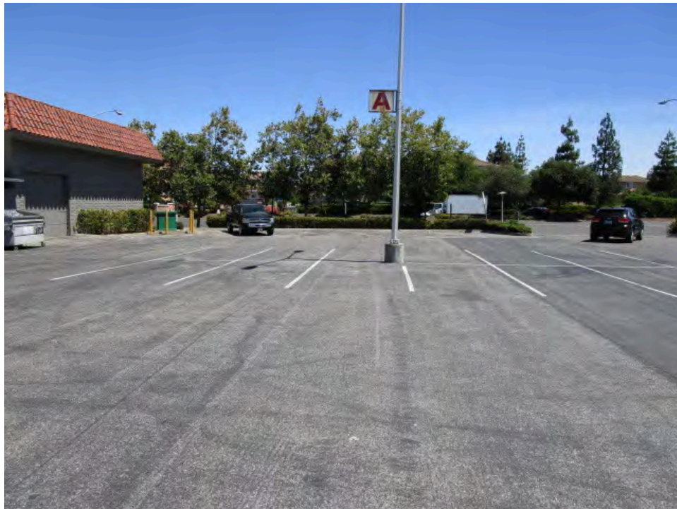
8. Asphalt-paved parking/drive area on the subject property
