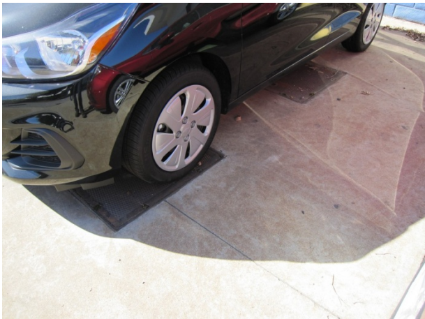
Photograph 25. Steel covers to oil/water separator at SAC.
