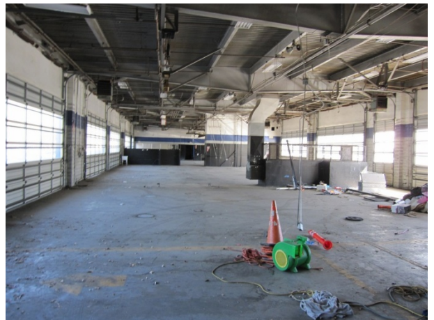
Photograph 16. Interior of SAC building.
