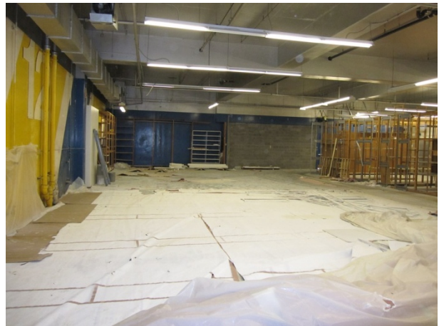
Photograph 26. Former auto service area at JC Penney.
