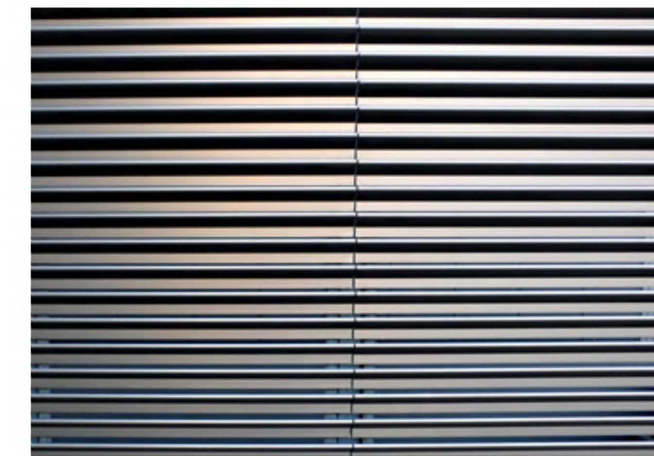
09 METAL LOUVERS 3/32" PAINTED ALUMINUM STORM LOUVERS BLADE
