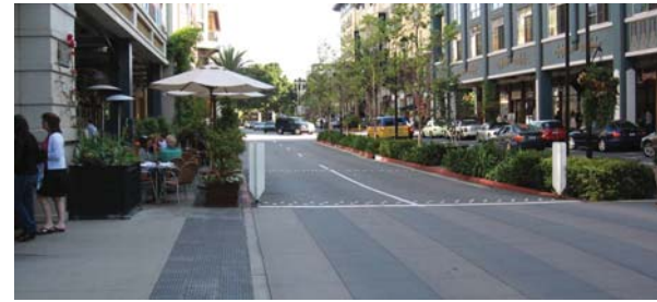
At-grade crossings with enhanced paving and detectable warning tiles for a safe pedestrian experience
