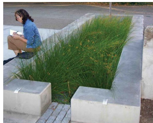
Seat walls at curbside rain gardens
