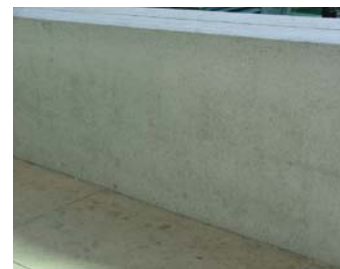
Cast-in-place concrete walls
