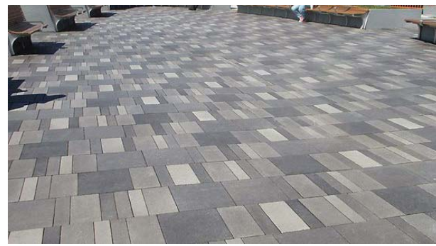
Concrete Pavers- various colors, textures, & sizes to compliment architecture
