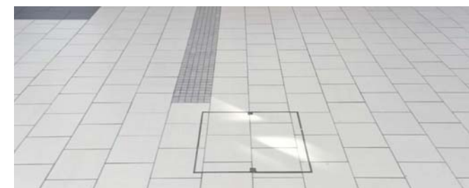
Utility vault lids to be infilled with concrete pavers or poured in place concrete
