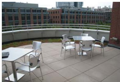
Concrete roof paver system
