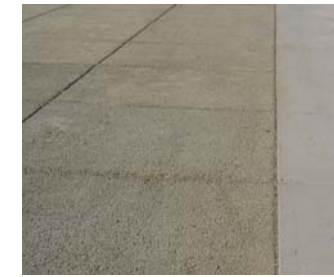
Porous Concrete at parking stalls, where feasible
