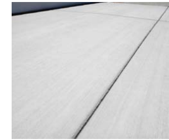
Basic gray, broom-finish concrete for City sidewalks
