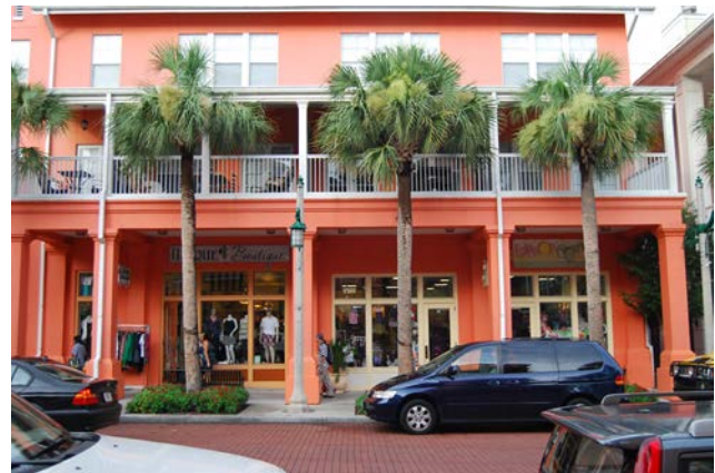
A two-story gallery with the second story covered.
