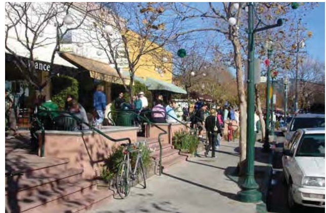
Terrace is used to accommodate a change in grade with low walls to provide seating.
