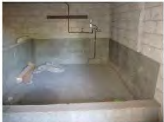
Photograph 28. Secondary containment area at JC Penney.
