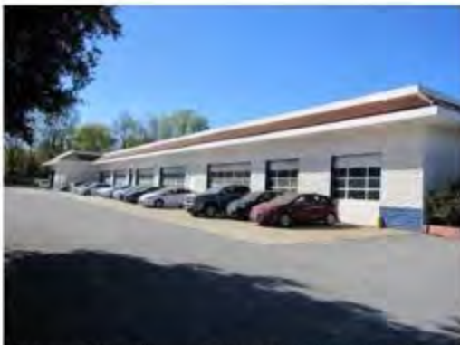
Photograph 15. Sears Automotive Center (SAC) building.
