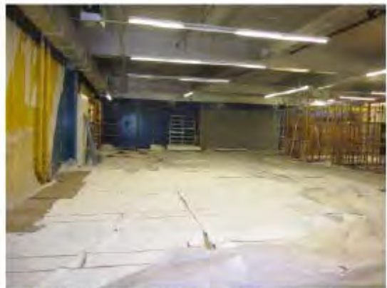
Photograph 26. Former auto service area at JC Penney.
