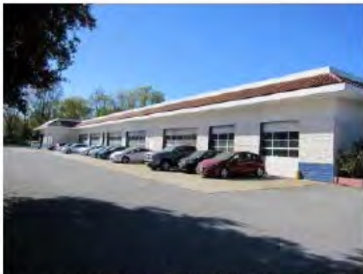
Photograph 15. Sears Automotive Center (SAC) building.
