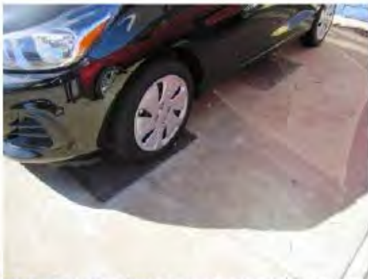
Photograph 25. Steel covers to oil/water separator at SAC.
