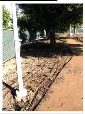
b. Option 2: "Six Inch Cover" Rule: Use a modified specification such as a setup where a maximum of six (6) inches of soil cover is specified as the maximum allowable vertical space between top of newly installed PVC irrigation pipe and original soil grade elevations, within 20 feet of a tree trunk. Below is a sample specification side cut detail showing this "shallow cut" type setup that was used for a recent project where new
