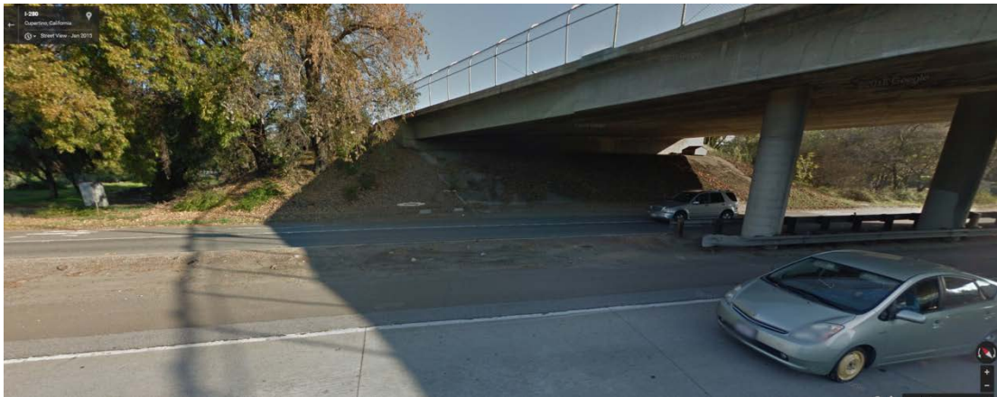
Figure 3-2 – View of west side (Wolfe southbound lanes) of Wolfe overpass from I-280
