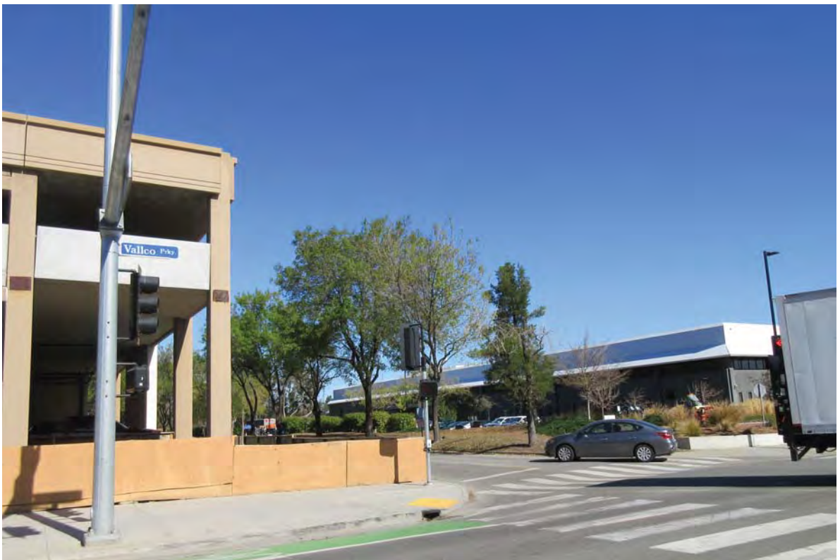
PHOTO 2: View of project site and adjacent office development from Vallco Parkway looking northeast.
