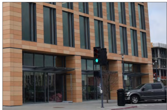
Shopfront with pilastered bays and recessed entry.
