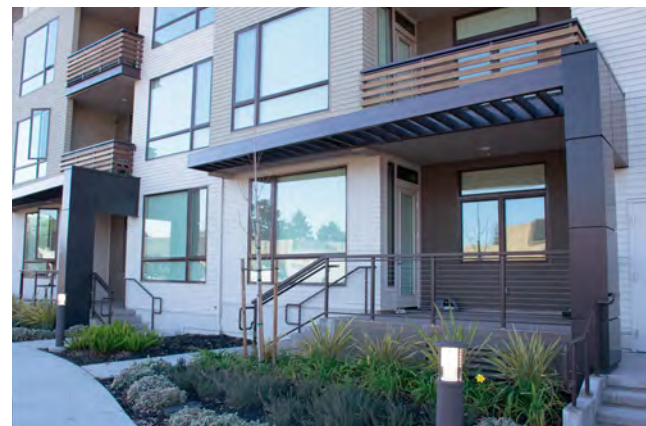
Example of projecting porch that extends the living area into the front yard.
