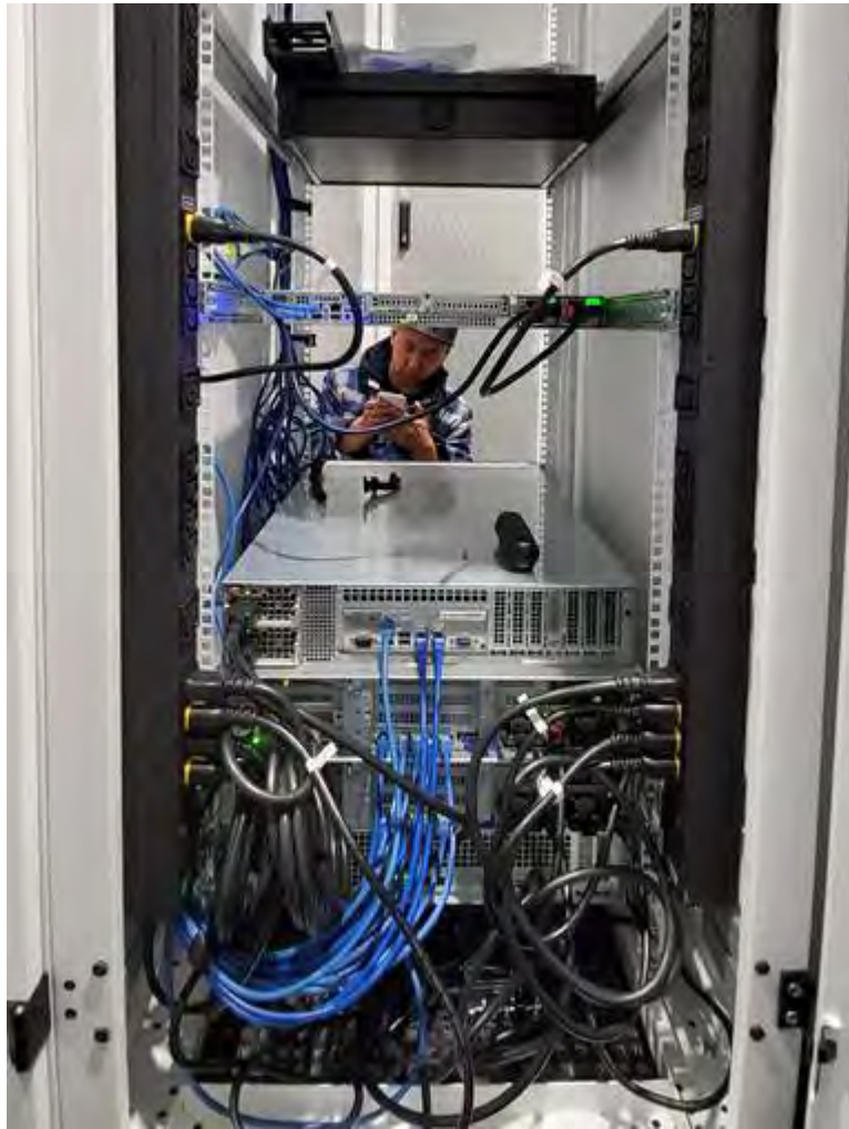
Phase 5: Toan verifying test results
