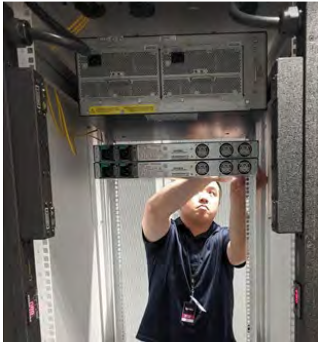
Phase 4: Benny installing Firewall protection within Cupertino's rack
