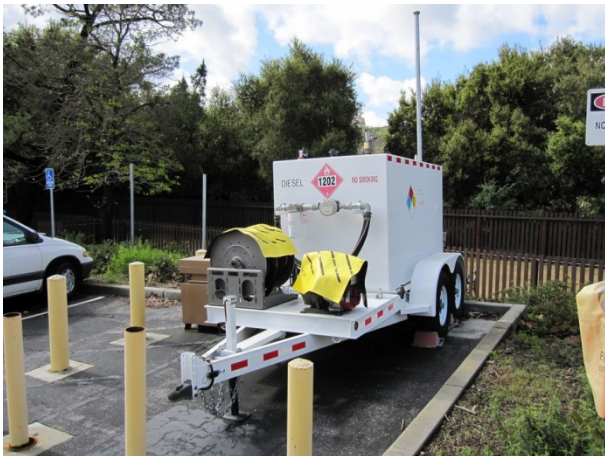
Photograph 5. 1,000 gallon diesel fuel AST.
