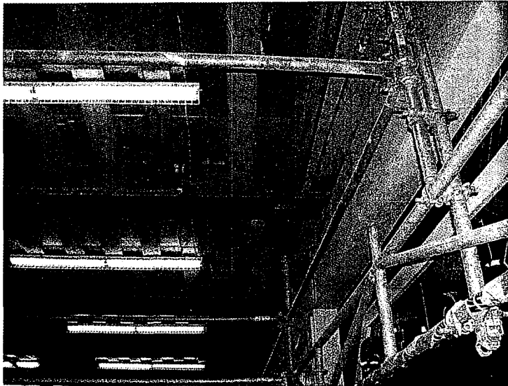
Photograph 8 - View of exposed infrastructure.
