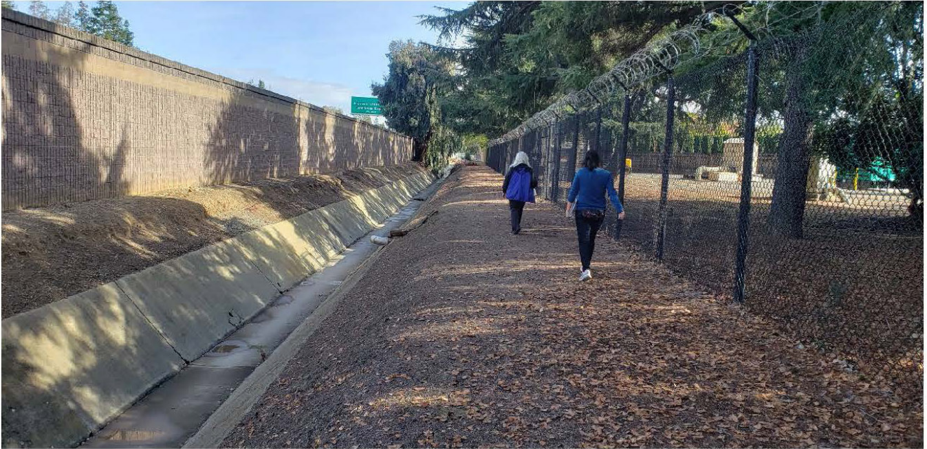
Photo 7. View of existing freeway soundwall and adjacent utility yard along the trail alignment. (Central section)
