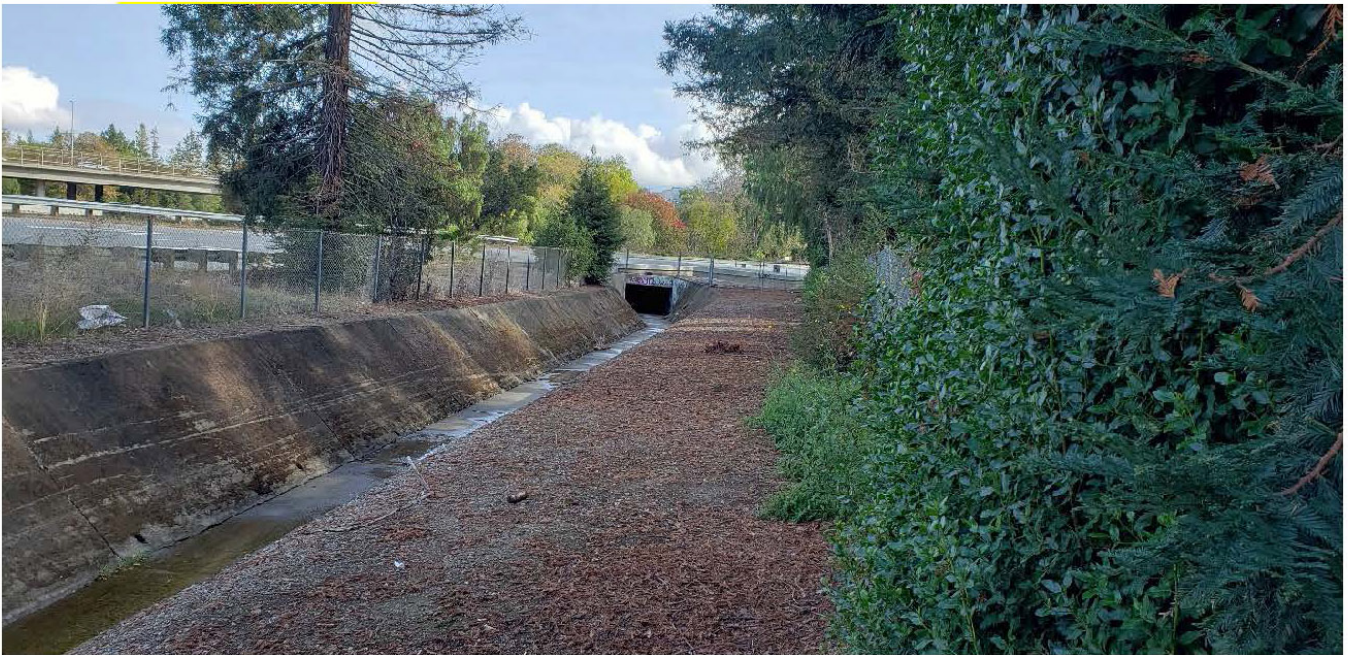
Photo 8. Viewing east along the trail alignment toward the SB I-280 offramp at Wolfe Road. (Central section)
