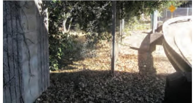
Pinch Point between Sound Wall and Guard Rail Figure 4-27
