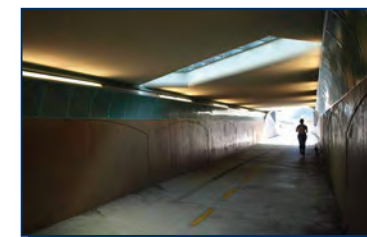
Tunnel Crossing Under De Anza Blvd.
