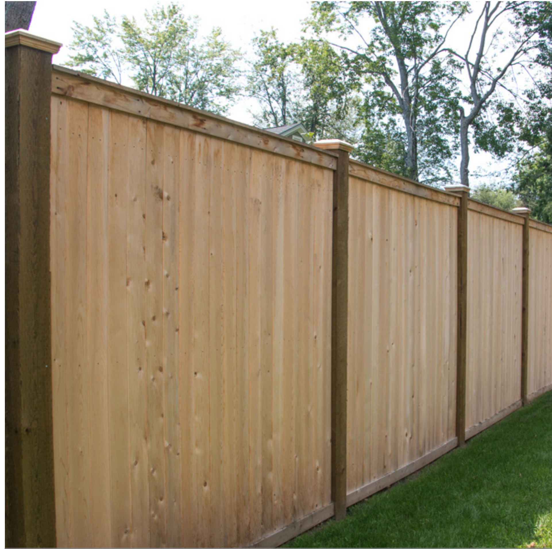
Privacy/Security Fence Adjacent to Residential
