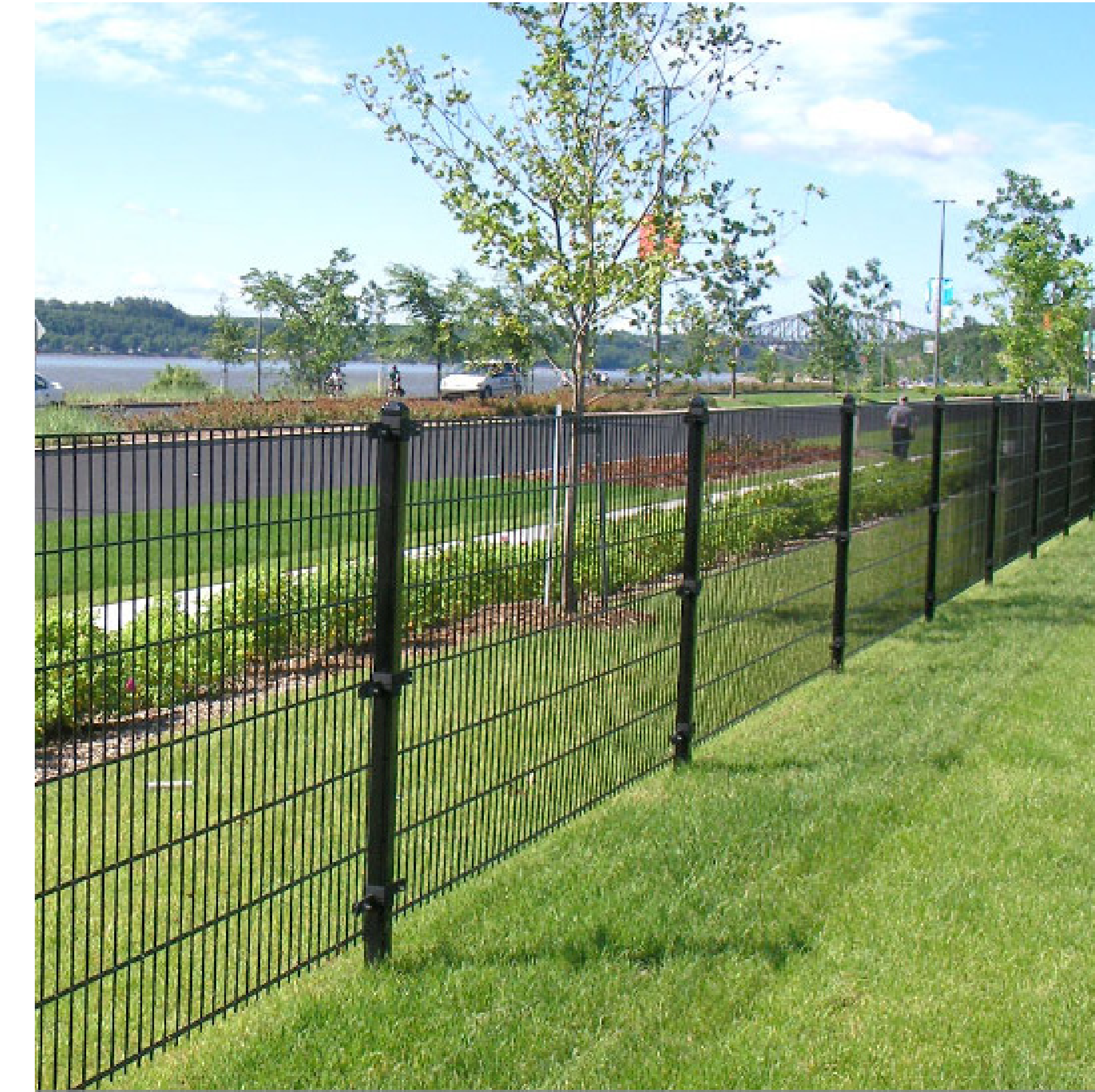
Guard Rail Adjacent to Open Ditch
