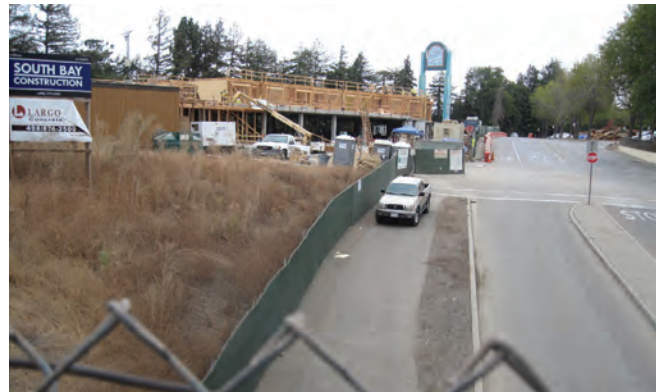
Hyatt Hotel House Under Construction
