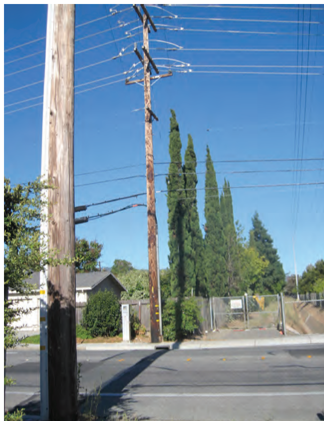
Existing Conditions at Stelling Road
