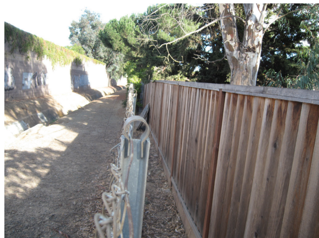
Fence Straddling SCVWD Corridor and Residences Figure 3-23
