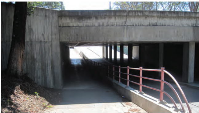
Underpass at Wolfe Road
