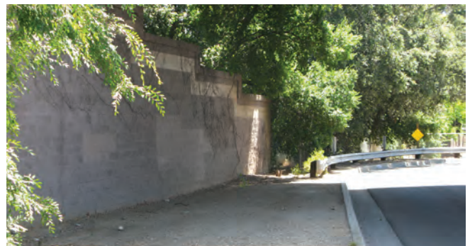
Existing Conditions below Blanney Avenue
