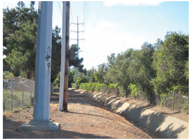
PG&E Utility Poles in SCVWD Corridor Figure 3-3
