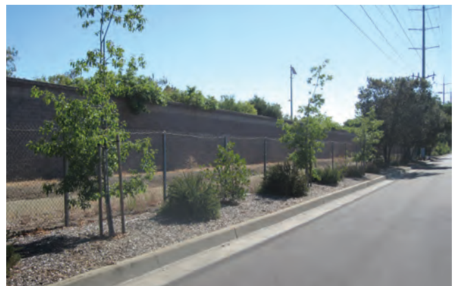
Existing Conditions along Lucille Avenue
