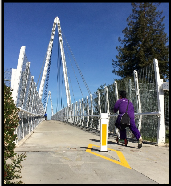
Don Burnett Bridge Bollard Replacement
