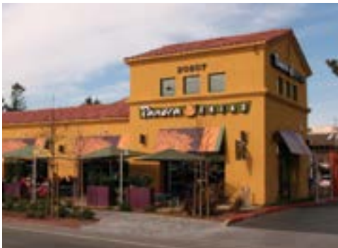
The North Crossroads Node is a key commercial/retail destination along Stevens Creek Boulevard and includes many newer, smaller scale stores and restaurants
