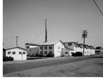
Woelffel Cannery 10120 Imperial Avenue Demolished
