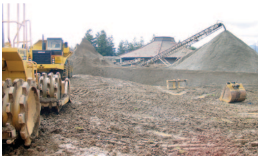
Recycled building materials used in Cupertino Library reconstruction
