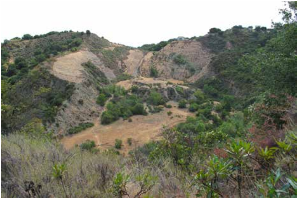
The steep cutslopes of the quarry are clearly visible.
